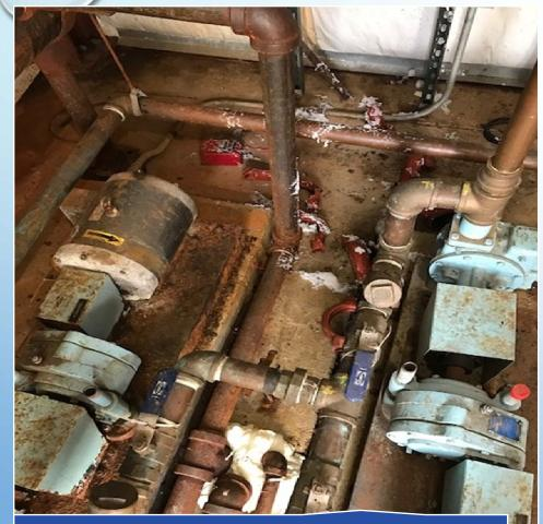
Foam residue and sealed off deck drain
